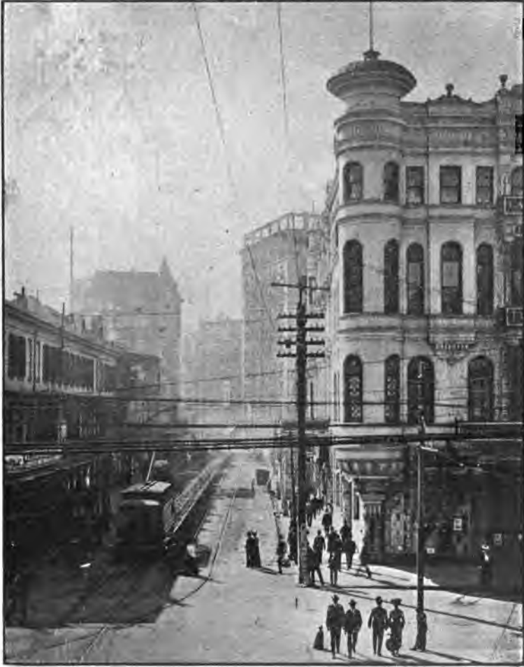
VIEW OF CARONDELET STREET FROM CANAL.
